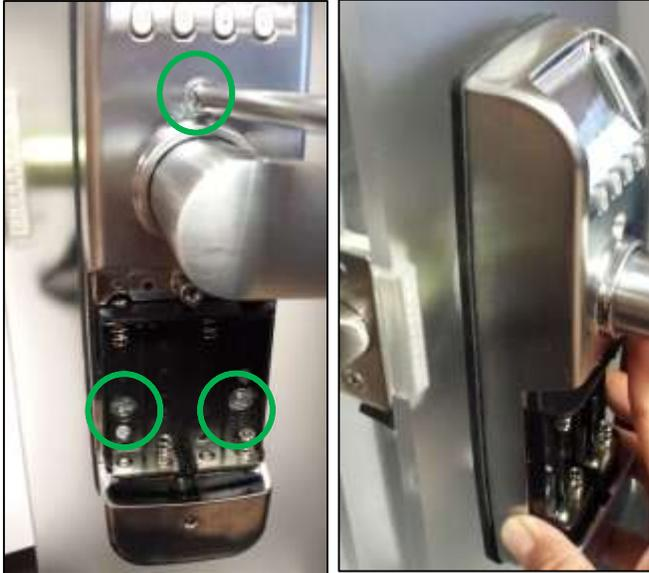
7) Affix lock to the door with the three screws from bag "D". The longer screw is for the top fixing post. The two shorter screws are for the bottom fixing posts.
