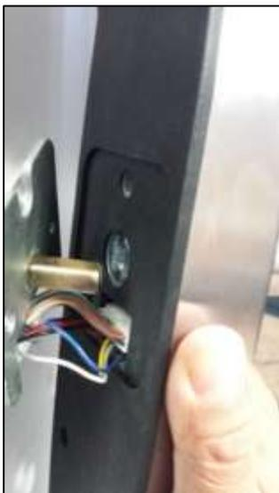
6) Push the excess cable and wires into the hole under the fixing plate.
