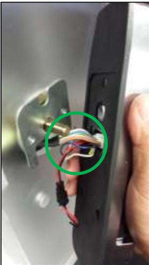
4) Feed the cable from the inside lock through the opening in the bottom side of the fixing plate.
