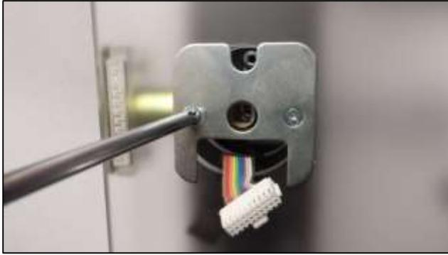
3) Screw the fixing plate onto the door with the provided 1 1/2" screws.
