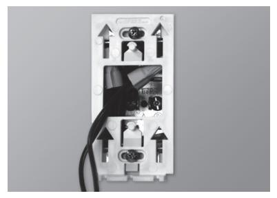
8. Align the little slots located on the top of the thermostat with those on the mounting base and secure the thermostat to the mounting base. Note that you can also position the thermostat on the left or the right side of the junction box (see the illustrations below). Then, tighten the screw at the bottom of the unit.
