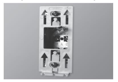
6. Pass the wires from the wall through the hole at the base of the mounting base and connect them using the supplied solderless connectors. When making the connection with aluminum wire, make sure that you are using connectors identified CO/ALR. Please note that the thermostat wires do not have polarity. Therefore, the way they are connected is not important.
