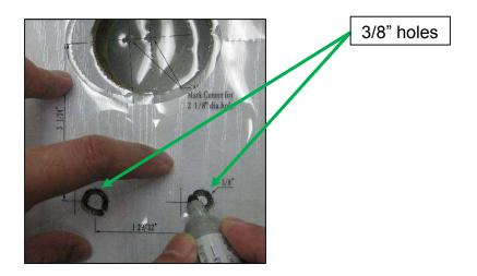
3) Now that you have the hole pattern marked on the template, use a utility knife to cut through the template so that you can mark the hole pattern onto the door.
